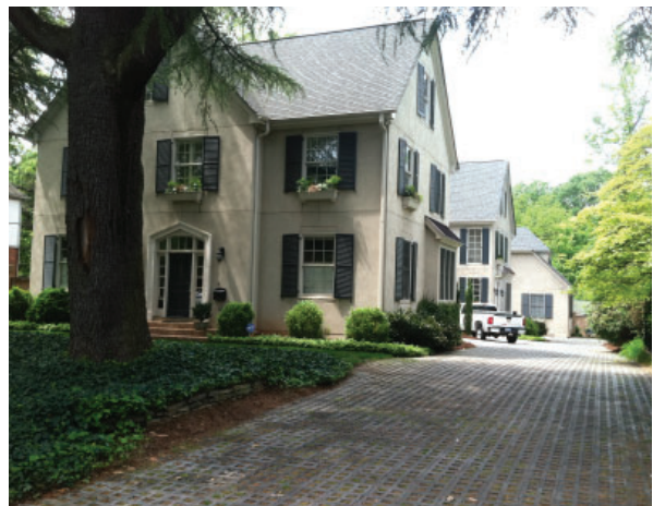
Actually, three units comprise this residential building. Each unit is accessible from the shared driveway and can accommodate parking for two cars per unit on site.
