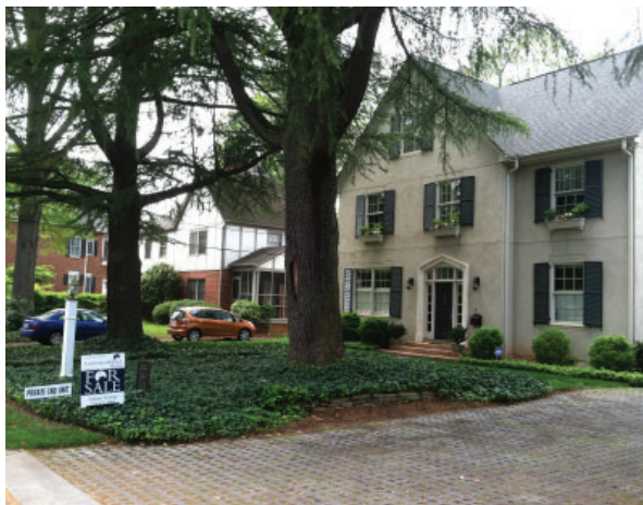
From the street, the structure has the appearance of a single-family home.
